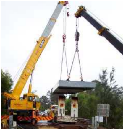
Figure 8 Coutts Crossing Demonstrator Bridge Deck During and After Installation
