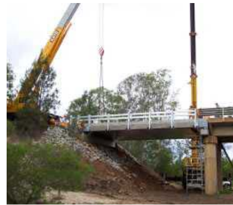
Figure 8 Coutts Crossing Demonstrator Bridge Deck During and After Installation
