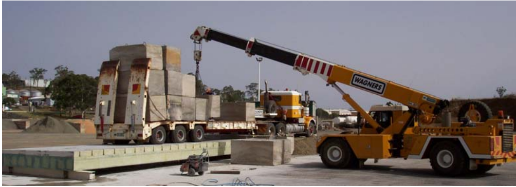
Figure 7 Proving Load Applied to Half Bridge Deck.
